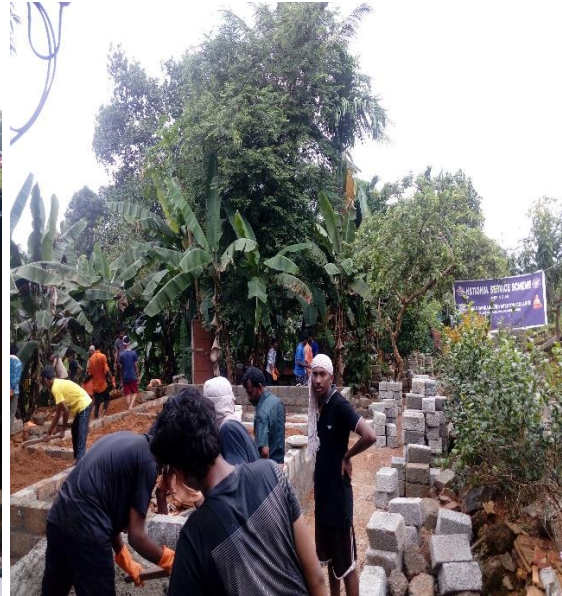
Work in Progress by Volunteers
